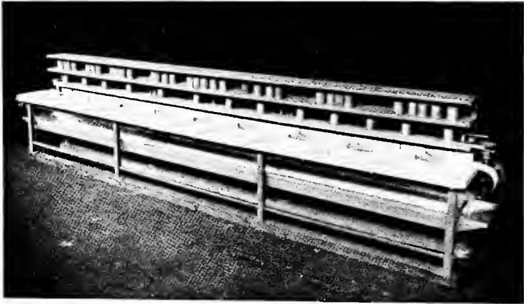
FIG. 11. Sanitary Canning Table
